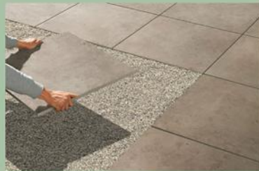
DRY LAYING ON SAND OR GRAVEL
