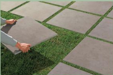
DRY LAYING ON GRASS
