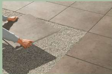
DRY LAYING ON SAND OR GRAVEL
