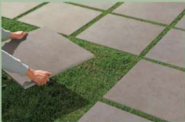
DRY LAYING ON GRASS
